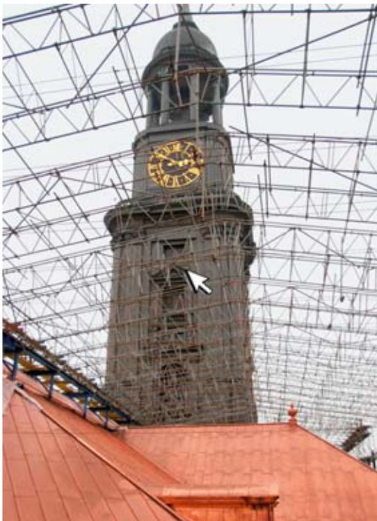
Aurubis provided 6,500 m 2 of copper for the Church of St. Michael in Hamburg and recycled the old copper
